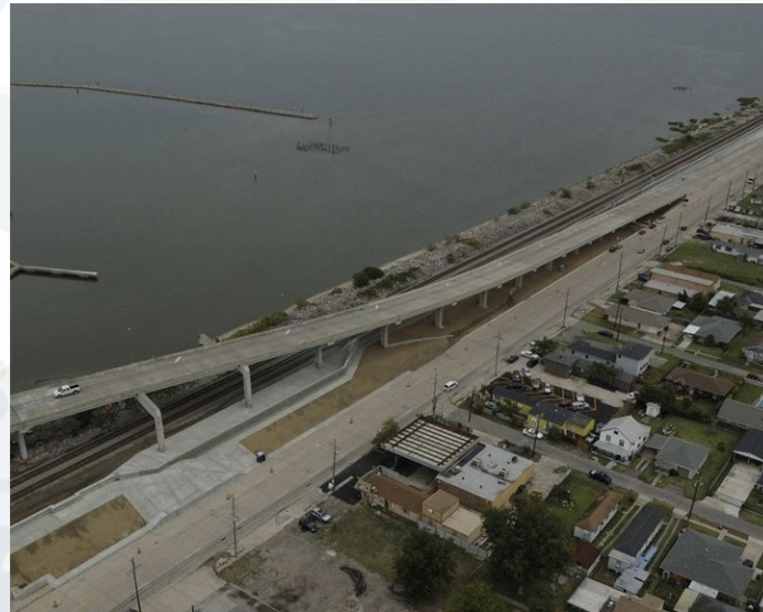
Build a flood wall
